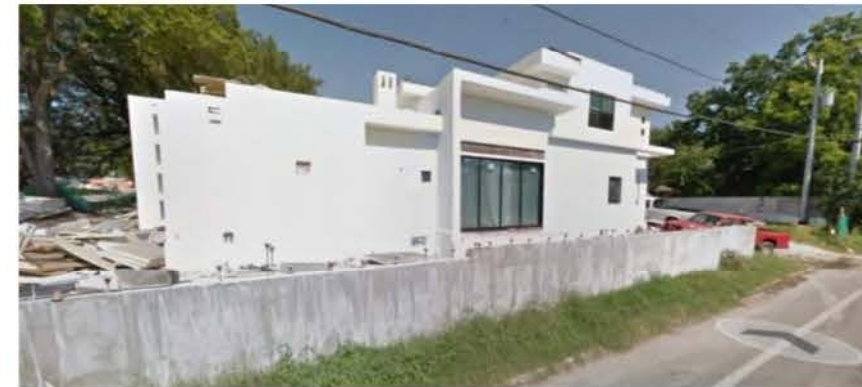
100 Canterbury Hill (Terrell Hills/Under Construction)
