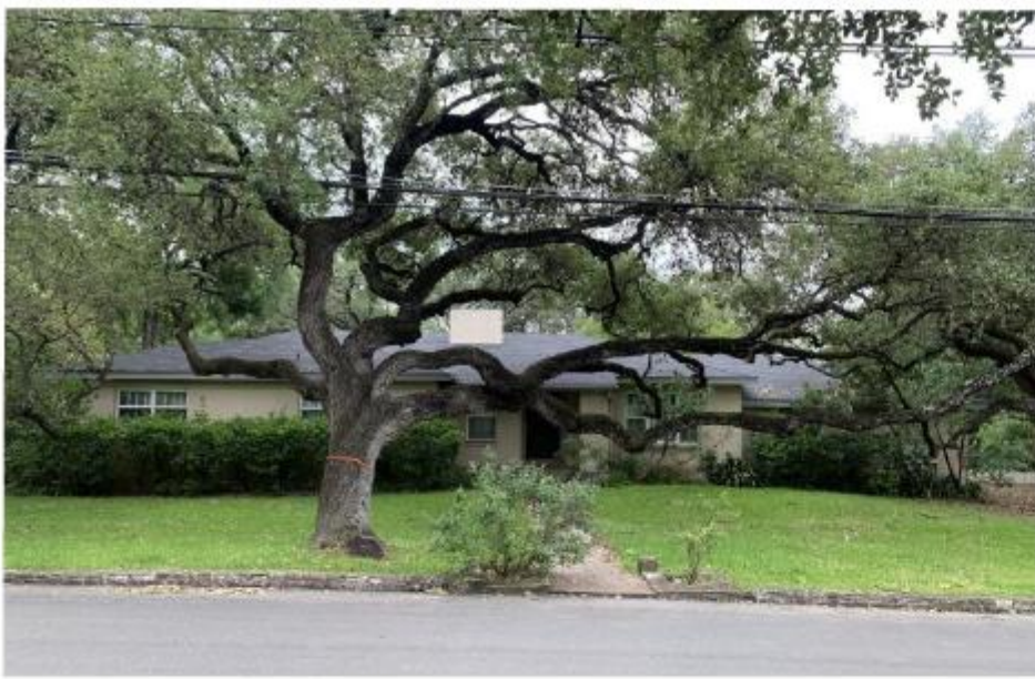
Front View of Existing House
