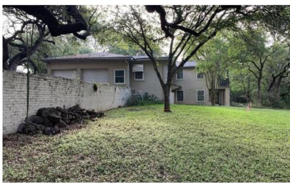
Left View of Existing House
