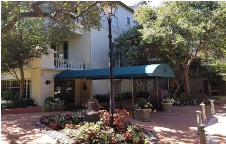
Existing Building Side View
