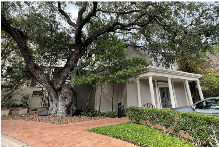
Existing Building Side View
