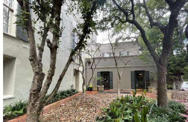
Existing Building Side View
