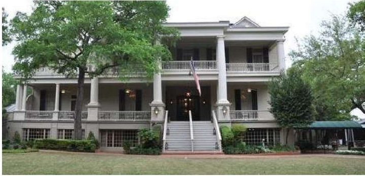
Existing Building Front Entry
